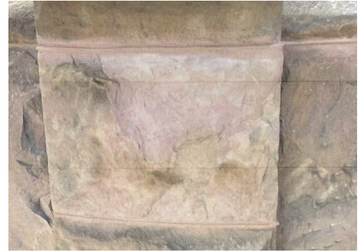
AFTER: Masons removed loose portions and patched to match stone.
