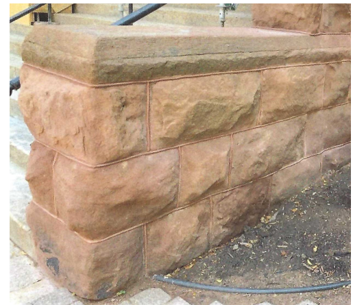
AFTER: Two stones replaced in wing wall, wing wall repointed.
